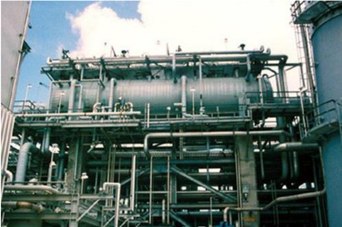
Horizontal drum at elevation on concrete foundation
