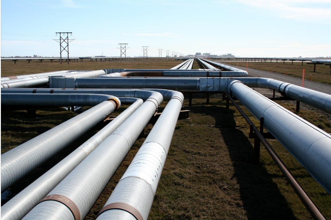
Expansion loops in aboveground piping.
